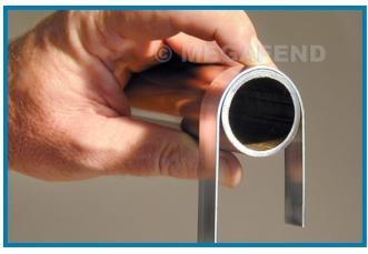
**Step 8**—(Pipe rails only) Bend metal strip or rod to shape of pipe rail. Measure I.D. to determine pipe rail O.D. for ordering.
